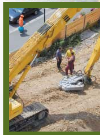
The demolition machine's quick coupler allows the mounting of a range of demolition processors and shears
