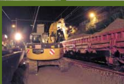
Positioned directly next to a passenger platform on its left, the PC128 is able to swing freely, without any worry of making contact damage.
