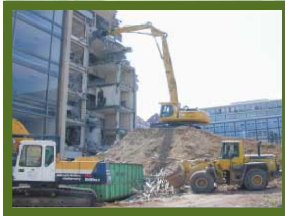
Working on a 6 m ramp, the longfront PC340-6 could reach the top of the building
