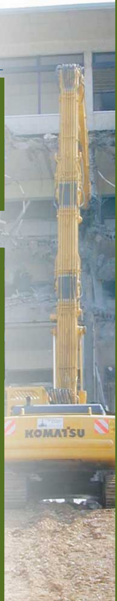
Working on a 6 m ramp, the longfront PC340-6 could reach the top of the building
