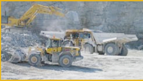
HD605-5, HD465-5, PC1100SP-6 and WA380-5 in operation
