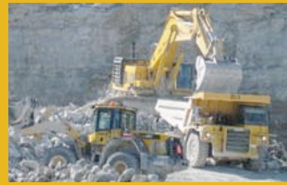
PC1100SP-6 excavator loading blasted limestone onto HD465-5
